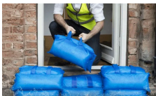
Temporary flood barriers
